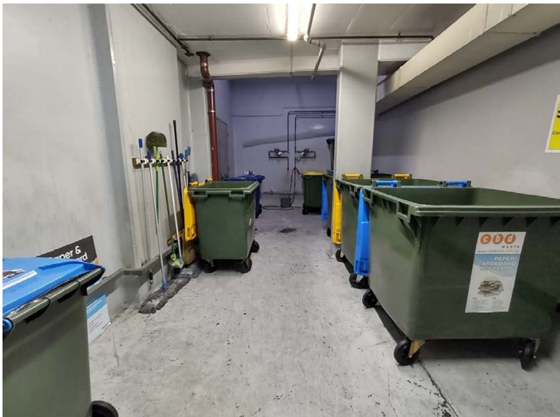
Photo 18: Recycled waste store room in basement 2
